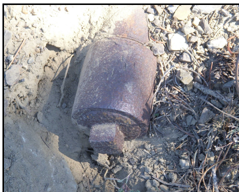
Fig. 3. Drain plug on the Prince of Wales pipeline is above the Silver Fork pass, where the pipeline turned north toward the mine.
