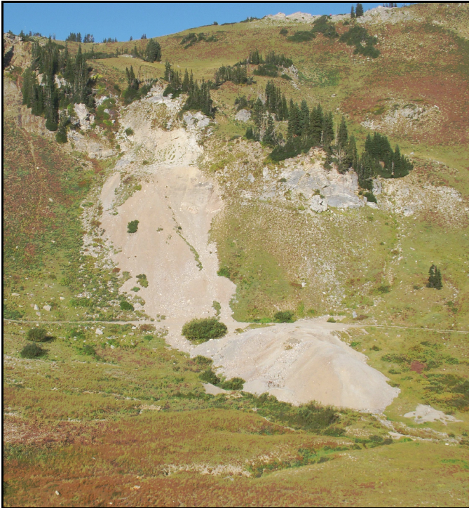
Fig. 1. The Albion mine as it exists in the upper southwest corner of Albion Basin. This was originally the Wellington mine of the early 1870s, with its shaft located at the top of the upper dump and its tunnel at the lower dump. An Alta Ski Lifts road now crosses the top of the tunnel dump, but the original Albion Mining Company road followed the same alignment. The flat in the foreground is the site of the early Wellington boarding house that was destroyed by an avalanche at the end of 1876.
