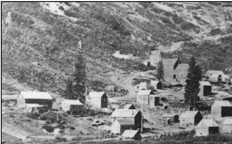
Fig. 2. The northern part of Alta city in late 1873, extracted from a Timothy O'Sullivan photograph. The large building to the right of center is the ore bin and lower terminal of the Vallejo aerial tramway. Two of the tramway towers can be seen on the hillside above the city. (Library of Congress photo)
