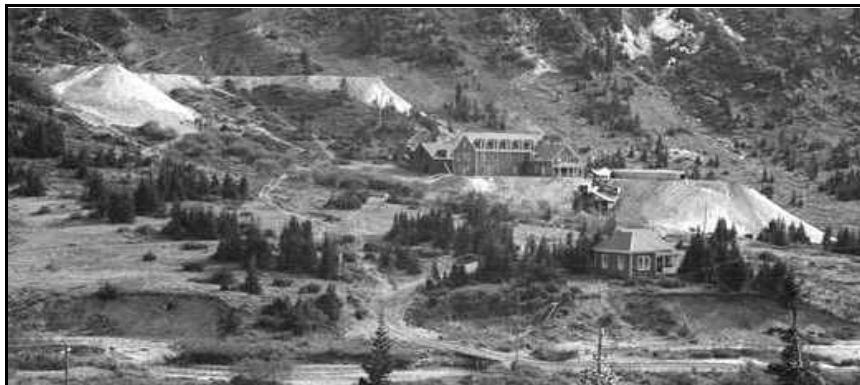
Fig. 2. This photo shows the South Columbus Consolidated Mining Company's base of operations as they appeared in August of 1915. By that time the South Hecla Mining Company had taken over the properties. The large mine dump at the upper left was from the Quincy tunnel, while the dump to the right of the three-story boarding house was from the Dwyer tunnel, whose portal was behind the buildings. The large compressor house is behind the boarding house, while snow sheds extend over the dump to ore bins and dumping areas. The building in the foreground overlooking Little Cottonwood stream was said to have been built for Tony Jacobson to use as his Alta summer residence.
