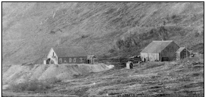
Fig. 2. This photograph, taken in the second half of 1904, after the Columbus Power Plant was operating, shows the boarding house and the big compressor house with its compressor driven by electric motors. The boiler and steam driven compressor have been removed. The faint line across the slopes above the buildings is the right of way for the old Alta horse tramway, later to be used for the Little Cottonwood highway. (Utah Historical Society photo)
