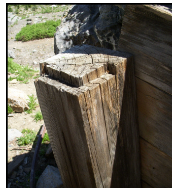
Fig. 3. Timbers at the portal of the collapsed Tarbet tunnel show the fine woodworking that went into mine timbering.
