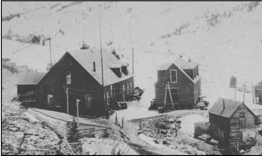
Fig. 1. These buildings survived the fire that destroyed the Columbus Consolidated boarding house in February 1913. They are, from left to right: the big compressor building behind the low barn, the office building with three dormers on each side of the roof; and a smaller two-story building whose purpose remains unknown. (University of Utah Special Collections)
