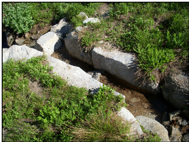
Fig. 3. Granite stonework provides a waterway across the trail to prevent erosion during spring snow melt, yet is narrow enough to allow man and beast to step across easily.
