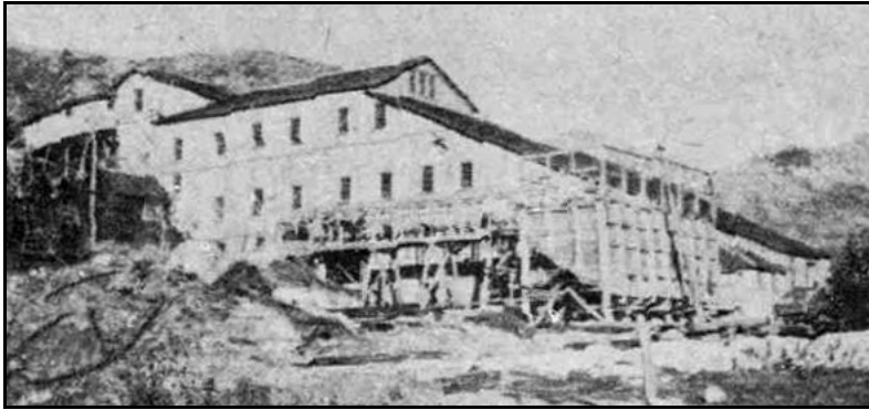
Fig. 3. Columbus Consolidated mill as it appeared during the later stages of construction, about August 1905. The ore bins at the front corner are not yet completed. A trestle, enclosed in a snow shed, leading to the portal of the Howland tunnel is seen behind the building at the upper left. The view is toward the northeast. (Salt Lake Mining Review photo)
