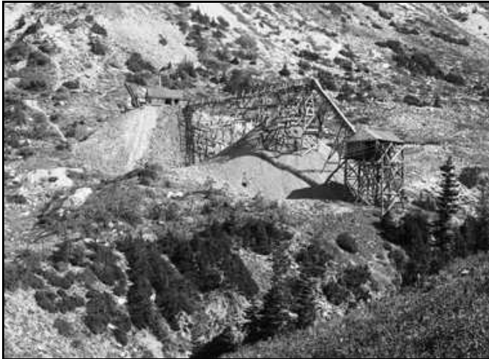
Fig. 3. The Alta Consolidated mine with its trestle, chute, ore bin and loading station as seen from the opposite side of Grizzly Gulch. The Michigan-Utah aerial tramway passed directly under the ore bin. (Utah Historical Society)
