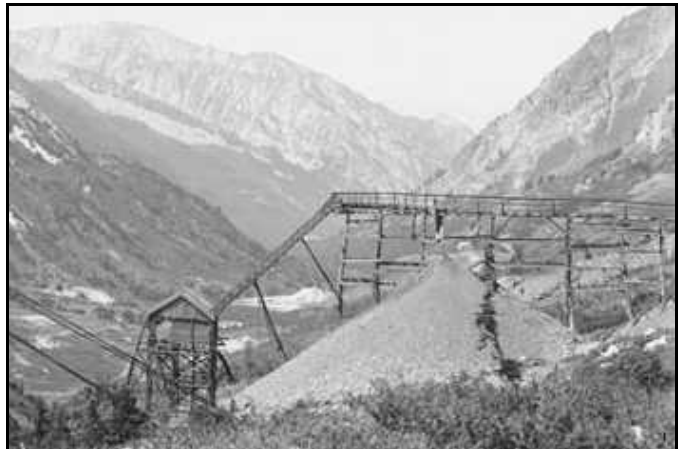
Fig.4. The Alta Consolidated trestle and loading bin. The view is looking down canyon, with Alta and Little Cottonwood canyon below. Notice the chute directly above the apex of the small mine dump that allowed waste rock to be dumped there. This photograph is dated 17 August 1915. It may be assumed the small dump was created during the year since June 1914, when the trestle was placed back into service. The cables in the lower left corner are from the Michigan-Utah tramway's upper terminal, contributing to its structural strength. The actual tramway cables ran under the Alta Consolidated's loading bin. (Courtesy Utah Historical Society)
