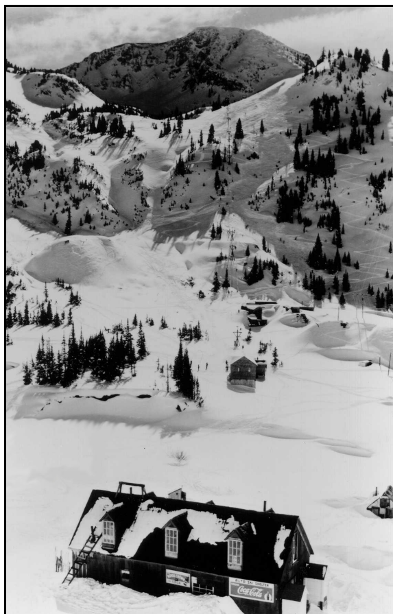
Fig. 2. The Red Shelter, formerly the office building of the Columbus Consolidated Mining Company. Notice the three dormers on each side of the roof. The base of the new Alta ski lift is across the bottom of the canyon. Collins Gulch is above and Mount Baldy is on the skyline.
