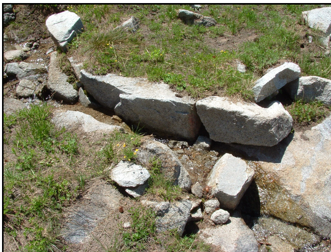
Fig. 4. Another granite gutter channeling water across to the other side of the trail, this one showing some of the ravages of time.
