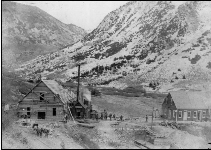
Fig. 1. This photograph, taken late in 1903, shows the large 35' x 80' building under construction to house an electrically driven compressor as well as a machine shop and blacksmith shop. It also shows the recently completed boarding house and the small steam driven compressor installed in 1902. The view is up canyon, with the south fork going off to the right in the distance. (Salt Lake Mining Review photo)
