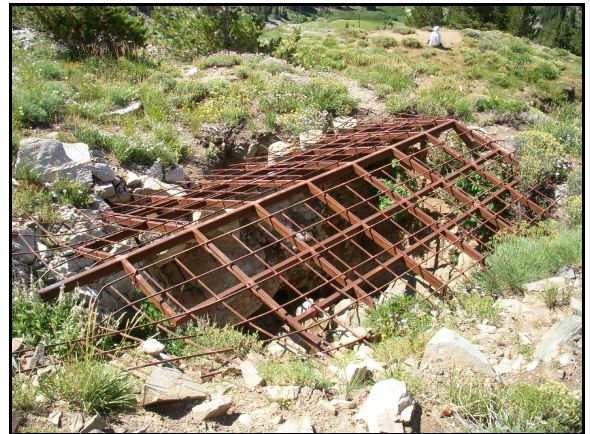
Fig. 4. A metal grate covers the open Marietta shaft. Below the far end of the grate the flat area that once held the Florinda mine cabin can be seen.
