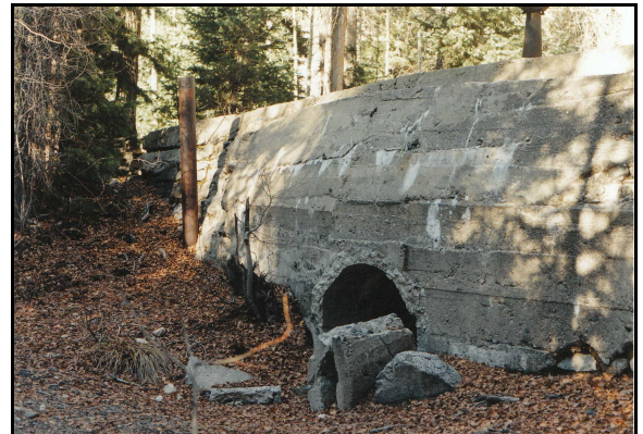
Fig. 4. This diversion dam diverted water from Little Cottonwood Creek into a 22-inch diameter steel pipe where it was carried to the power plant about 4,500 feet away. The dam is located at the lower end of the Tanner Flat campground.
