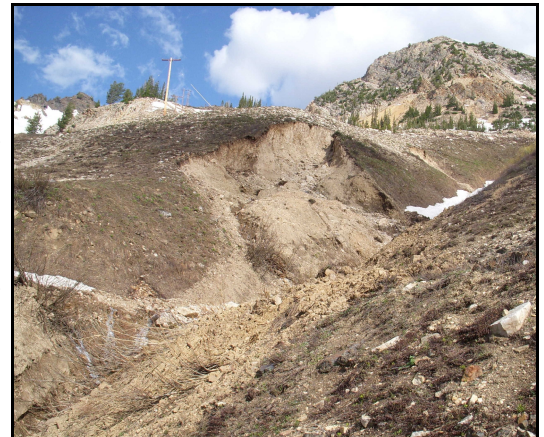
Fig. 4. A massive collapse of the hillside on the west side of Emily Gulch occurred in the spring of 2010. The Toledo Tunnel on the Michigan claim is located at the left side of the photo, about the same elevation as the collapse.
