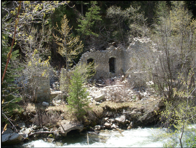
Fig. 3. The sad remains of the Columbus Power Plant as seen in May of 2012. Except for a portion of the rear and west end wall, there is only a pile of stone where the once proud building stood. The tail race conduit for the east generator now sags into the stream.
