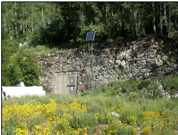
Fig. 4. The massive stone wall built by Martin K. Harkness in 1885 still stands at the portal of the Frederick Tunnel, now closed by a substantial door.
