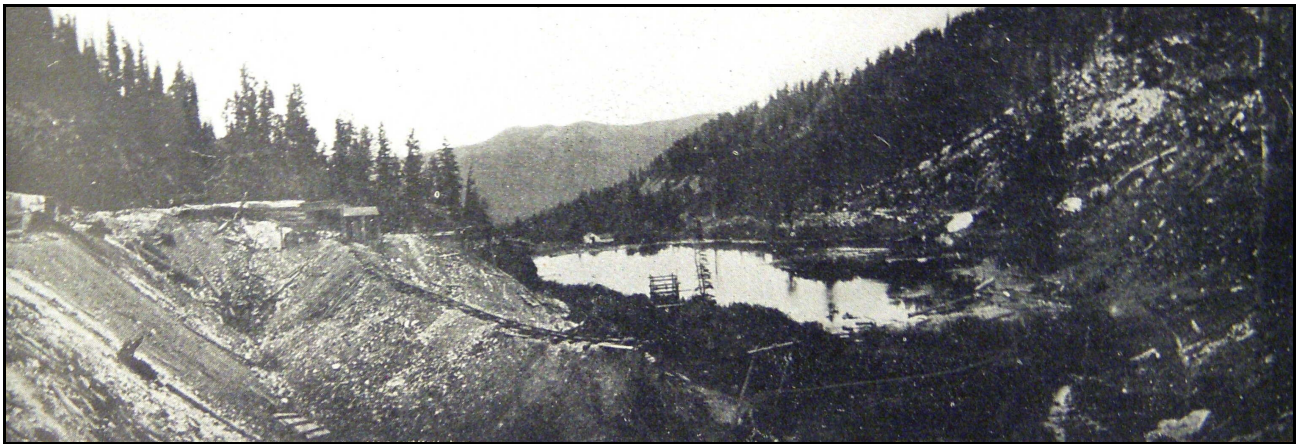
Fig. 3. Lake Solitude with the Solitude Tunnel on the left, as it appeared around 1913. (Salt Lake Mining Review)
