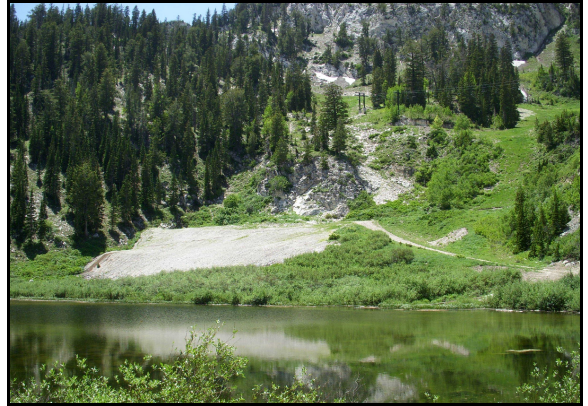
Fig. 1. The remnants of the dump at the Solitude Tunnel rise on the other side of Lake Solitude..
