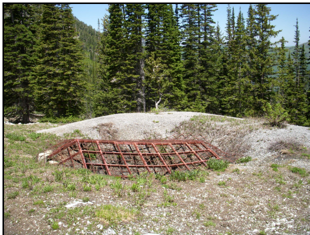
Fig. 3. The Gypsy Blair shaft, located above the Days Fork trail about 2.8 miles from the Big Cottonwood highway, is protected by a substantial metal grate.
