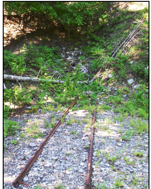
Fig. 2. The Victory Lode Mining Company's collapsed tunnel with rails extending out on the dump.
