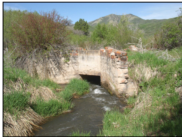
Fig. 3. An abandoned stone and concrete bridge of the early Parleys Canyon highway remains about a fifth of a mile east of State Highway U-65. The two summits on the skyline are on the ridge between Parleys and Emigration Canyons.
