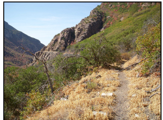
Fig. 4. View looking west along the Granite flume trail. Concrete foundation blocks from the 1931 reconstruction can be seen on each side of the foot path.
