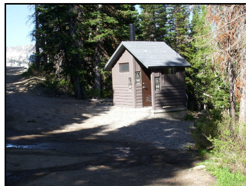
Fig. 2. A brilliant light from the heavens shines on this quaint U. S. Forest Service structure built on the old Scotts Pass road.
