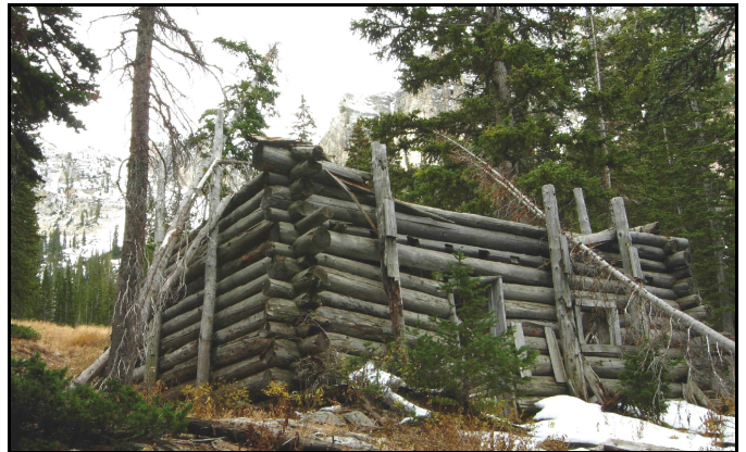
Fig. 5. Remains of the boarding house in the woods a short distance above the Woodlawn mine, as it appeared in 2006. (W. Nelsen photo)
