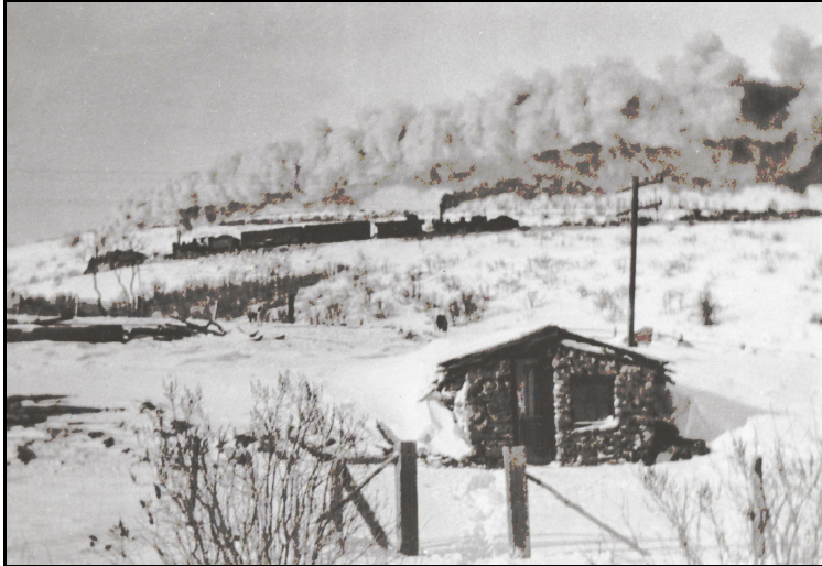
Fig. 2. Three Utah Central locomotives on a Parleys Canyon grade, possibly at or near Mountain Dell. (Author's collection)
