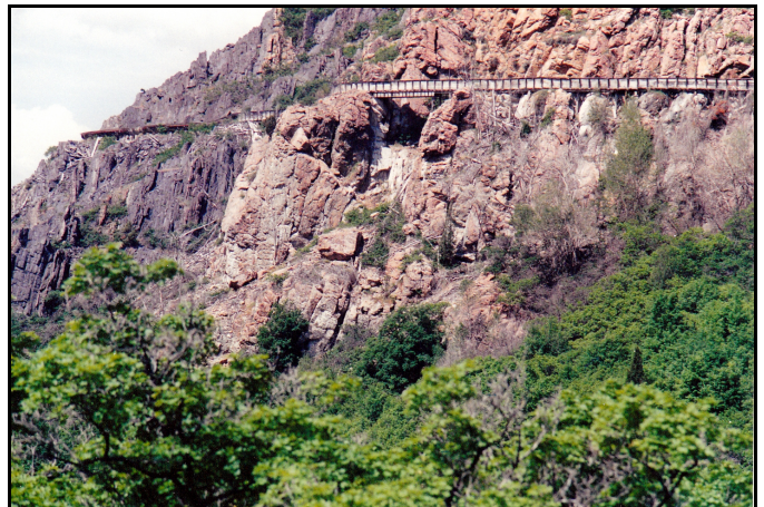
Fig. 2. This is the Granite Power Plant flume as it appeared high on the north side of Big Cottonwood Canyon.
