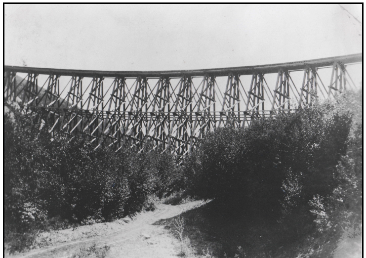
Fig. 3. Lambs Canyon trestle on the Rio Grande Western Park City Line. Built in 1898, it was about 300 feet long on a curve and 82 feet above the creek. (Utah Historical Society photo)
