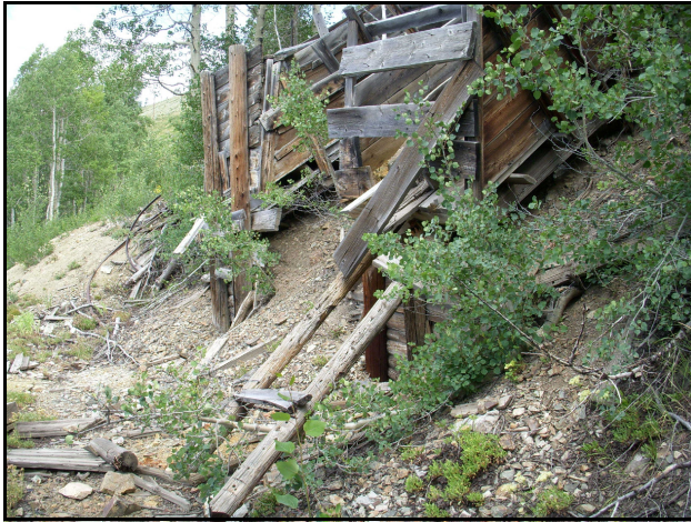
Fig. 3. Two ore bins are found below the road to the Scottish Chief mine. While they are below the Copper Apex workings, it is believed they were also used to hold Scottish Chief ore.
