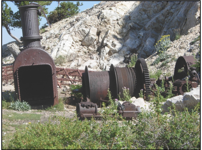
Fig. 1. Boiler and winch at the Prince of Wales mine in Silver Fork. The framework in the background is a protective cover over the inclined shaft that is at least 700 feet deep. (Wm. Nelsen photo)
