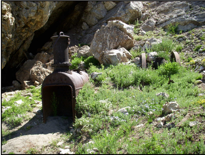
Fig. 2. Boiler and compressor at the Wellington tunnel. The tunnel, in the background behind the boiler, has suffered considerable collapse over the years.
