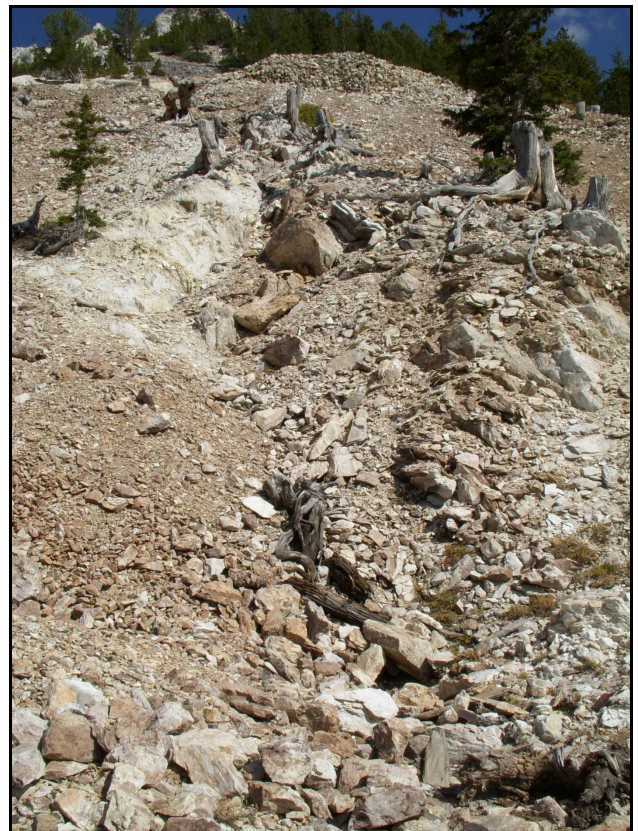
Fig. 5. Collapsed Prince of Wales tunnel, located along the lower road below the Prince of Wales boiler site. What appears as a stump or remnants of a tree at lower center is actually cribbing, a retaining wall that held back soil at the portal of the tunnel. The stone wall at the top of the photo supports the flat at the boiler and winch. The discovery incline, halfway up the slope, is no longer visible.
