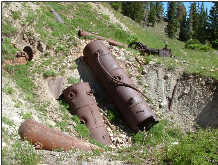
Fig. 3. Boilers sinking into the collapsed shaft at the Eclipse mine. The tank in the foreground was for compressed air. Machinery rests above and behind the shaft. The flat area in the background held the buildings for shops and miner housing. They were built against the bank on the left so the roofline merged with the slope of the hill above.
