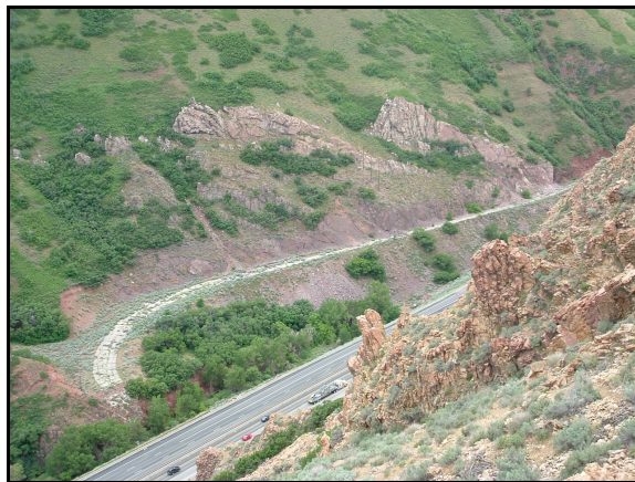
Fig. 3. Original Wasatch Boulevard running up canyon to the Stillman Bridge site on the south side of Parleys Canyon. I-80 is directly below.
