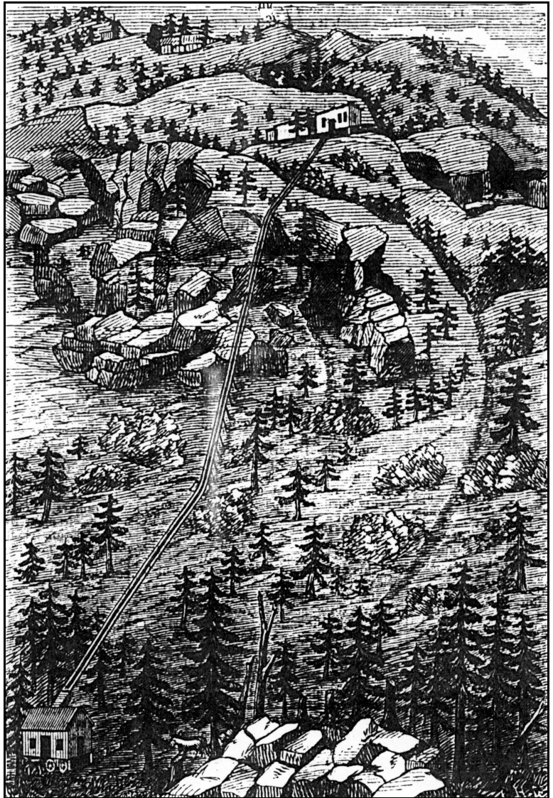
Fig. 3. The only known view of the Reed and Benson tramway is this artist's sketch published in the Utah Mining Gazette of 13 December 1873. Notice the houses on the ridge, an indication of miner's cabins, some of whose stone walls can still be seen on the Reed and Benson ridge a short distance north of Flagstaff Mountain.
