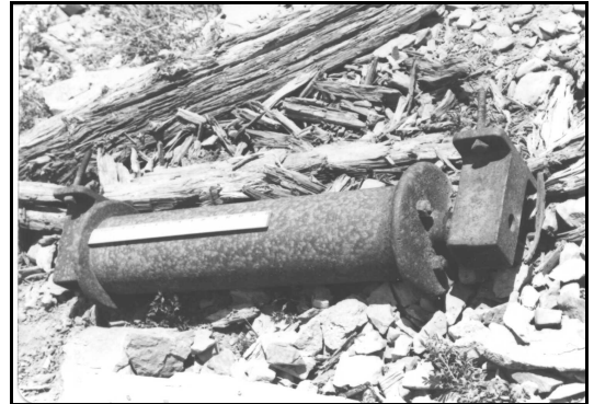
Fig. 3. The roller was bolted to the top of the lower cross arm, one at each end to support the moving hauling cable. A twelve-inch ruler gives an indication of the roller's size.
