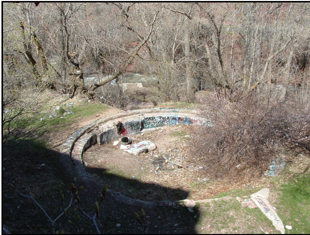
Fig. 2. Top of the settling tank on the northwest side of Suicide Rock, with the concrete base for the conduit leading to the stream below.
