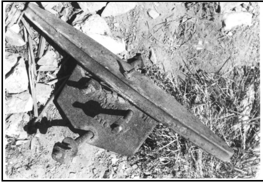
Fig. 2. Carrier casting bolted onto tramway tower upper cross arm to carry the large cable.
