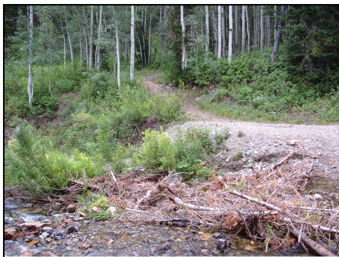
Fig. 3. The ford where the road crossed the South Fork stream. The old Reed and Benson road went down through the vegetation on the left, dropping to its ford. A newer road was built on a lesser grade to cross a ford on the right, above the old one, which has washed out badly since it was first used. This is at point E on the map.
