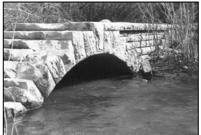
Fig. 3. Part of the beautifully executed stone arch bridge that carried the water conduit across Parleys Canyon creek. This photo was taken in 1972.
